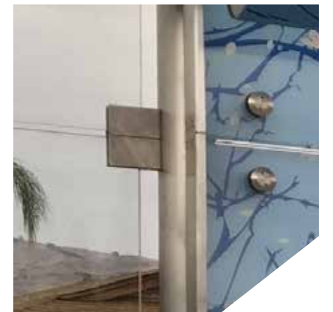
Deadload Clipz are shown on the left with glass bolts shown on the right.
