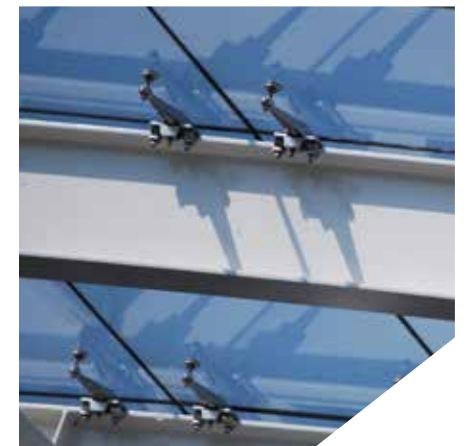
Wide-Arm clamps and steel structure shown
