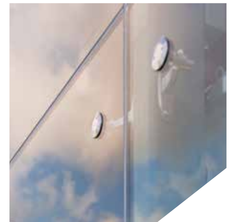
View from the exterior of Inlet Centre Station Line (Coquitlam, BC)
