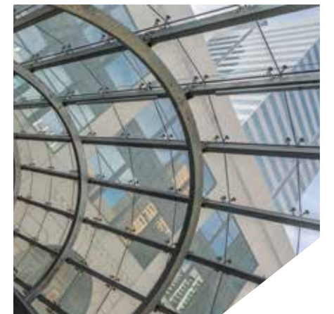
Faceted Glass Canopy West 7th LRT Station
