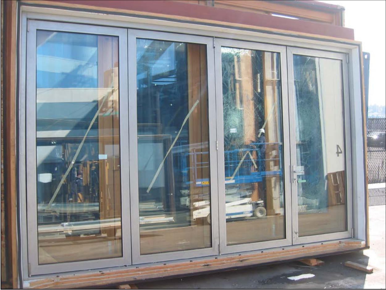
Photograph No. 1 – Exterior View
