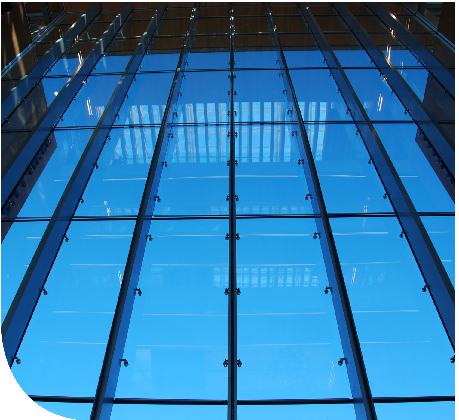
Structural Glass Wall, Surrey Civic Centre - Surrey, BC
