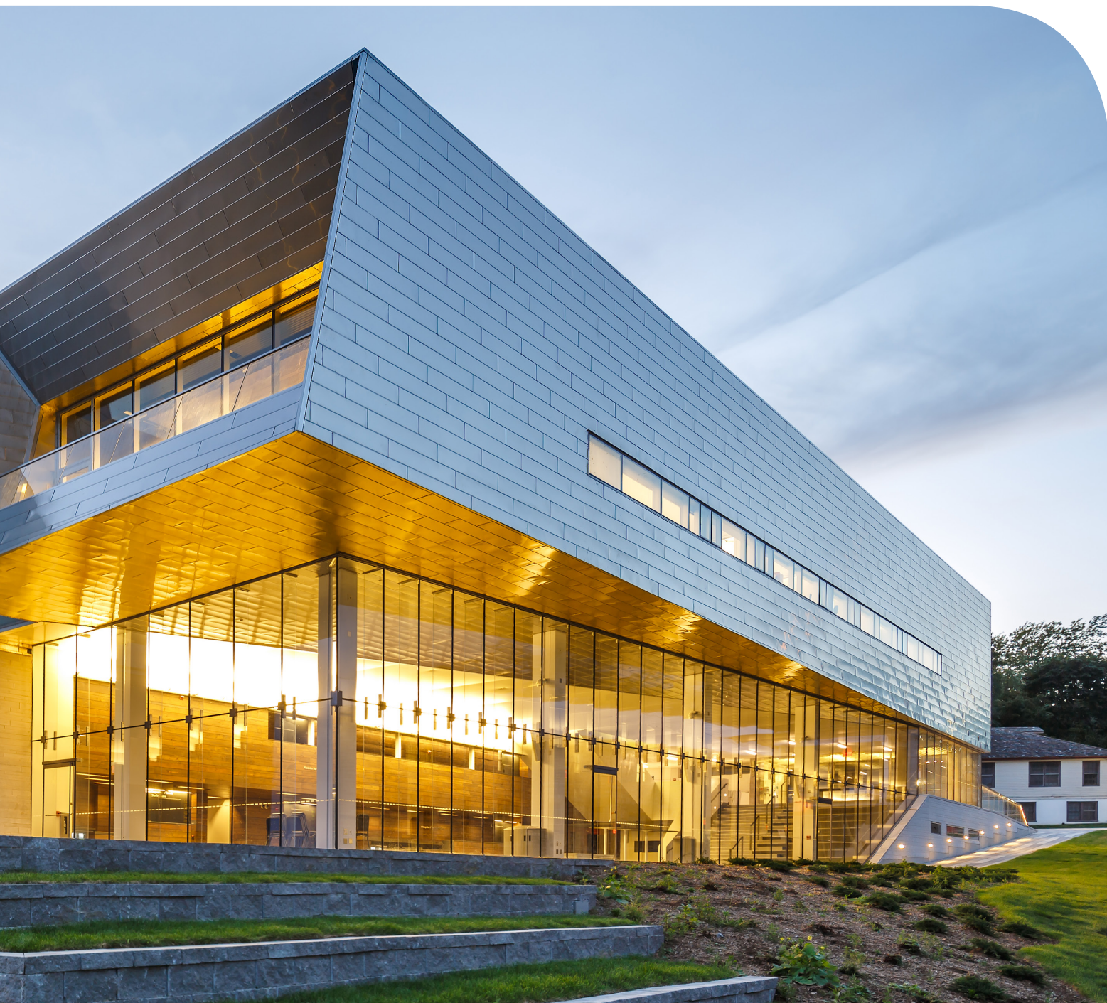
Structure Glass Fin Wall, Isabel Bader - Kingston, ON
