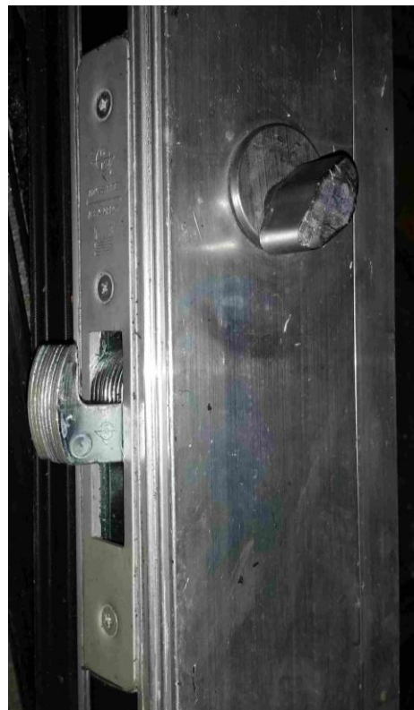
Figure 37 – Locking assembly
