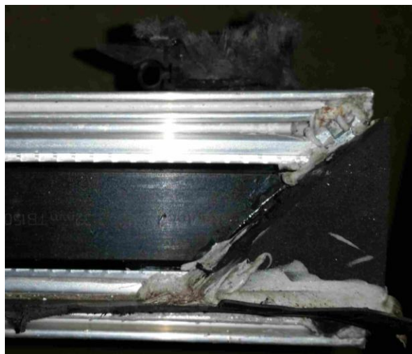
Figure 22 – Triangle shaped foam gasket on top rail of sash
