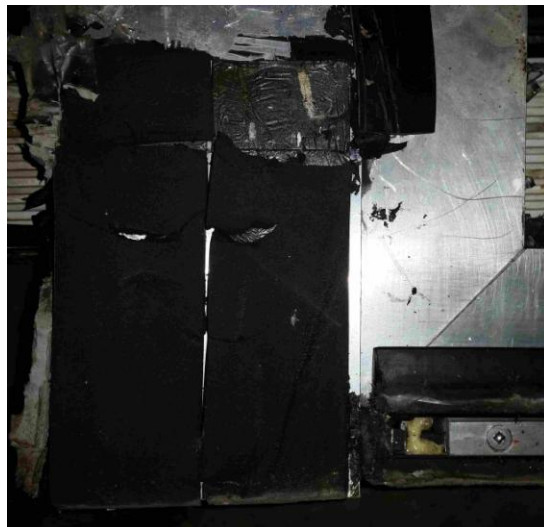
Figure 21 – Foam gaskets used above sash interlock
