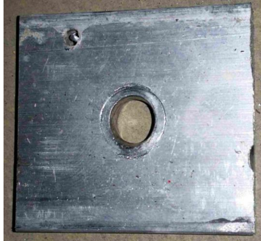
Figure 36 – Aluminum plate inside top rail to secure roller assembly
