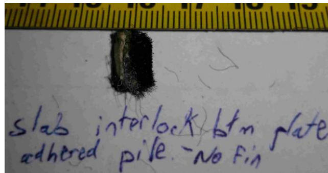
Figure 30 – Adhesive pile weather-stripping on the aluminum plate at the bottom of sash
